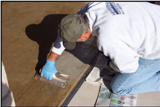
4. Fill / Repair Prepped Areas
