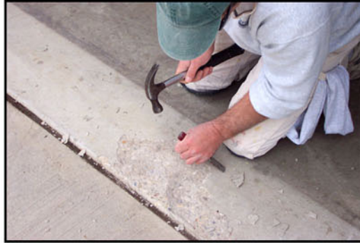
2. Scrape and Remove Loose Areas
