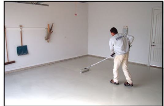
6. Apply 100% Solids Epoxy Coating
