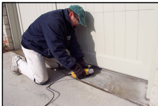
5. Smooth Repaired Areas
